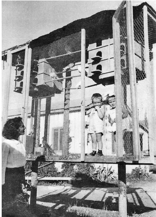
Ventilation pipes of the radio room are the base of the Dovecote 1943 photograph, courtesy Haganah Historical Archive
